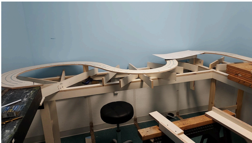
The roughed in base of Horseshoe Curve.
