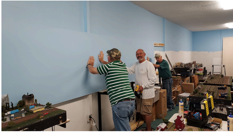
Extensive prep work was done before and during the rebuild.
