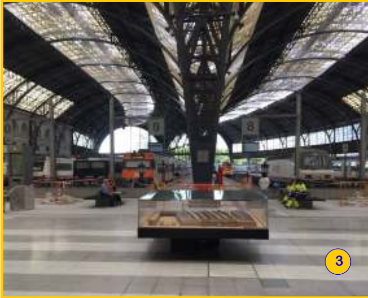
The train shed at Estacio Franca.
