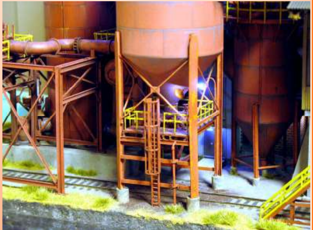
Photo 4 Detail of the base of the dust catcher. The structural element between the four legs with the yellow railings is a pug mill in which the dust from the stack is moistened and concentrated. Doug sells a resin kit for the basic pug mill but you have to supply the piping, valves and railings. He also beefed up the dust catchers' legs.
