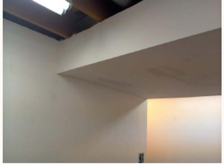
Soffit surrounding the air duct
