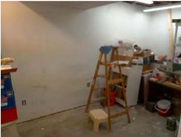
Walls where the shelves used to be
