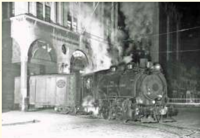
B&O C-16 0-4-0 switching Baltimore News Post Building—1940s
