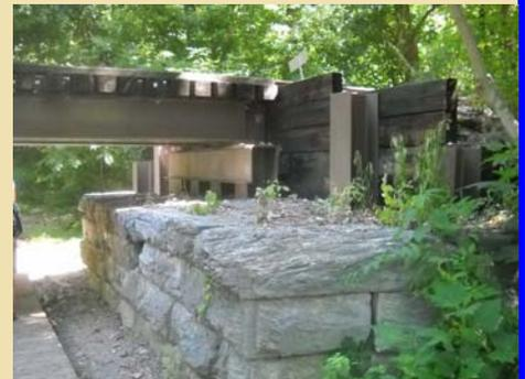
Even though the 3 bents are made of the same 14-inch I-beam legs with 2 opposite facing 18-inch tall U-beams and a 16-inch welded cap (Figure 2525), the trestle has two different ends. The east end (closest to Harpers Ferry and the Main Line) has its original cut stone pier there. Whether the new pier was driven in or the stones were removed and then reinstalled, I don't know. The stone pier walls are 24 feet wide and 7 feet deep, approximately 4 feet high.
