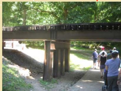
The trestle 45 feet long with a bent supporting the middle and one at each end with a wooden retaining wall to hold back the roadbed. The beams are each 22-1/2 feet long and are welded together on top of the center bent.
