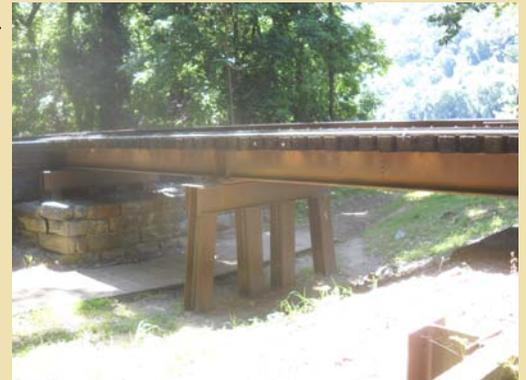
The walkway under the right hand/east side is 32 feet long and 8 feet wide. It appears to be just pressure treated wood but is not stained or painted. The top planks are 2 x 6 inches. There are 4 stringers underneath. The outer two are set in 6 inches; the inner two are then 2-1/2 feet further in. The planks are attached to the stringers with nails. The walkway is actually built in two sections since the ground slopes down from both side to a low point under the bridge.
